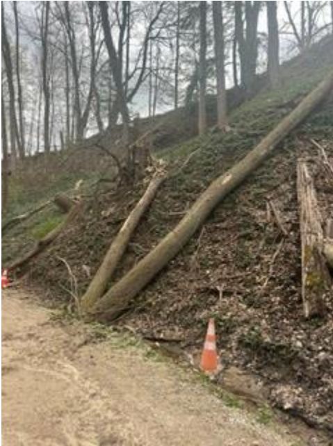
Tree damage and impact
