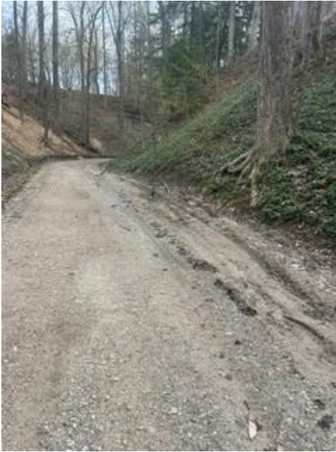
Wash out of trail and debris in swale
