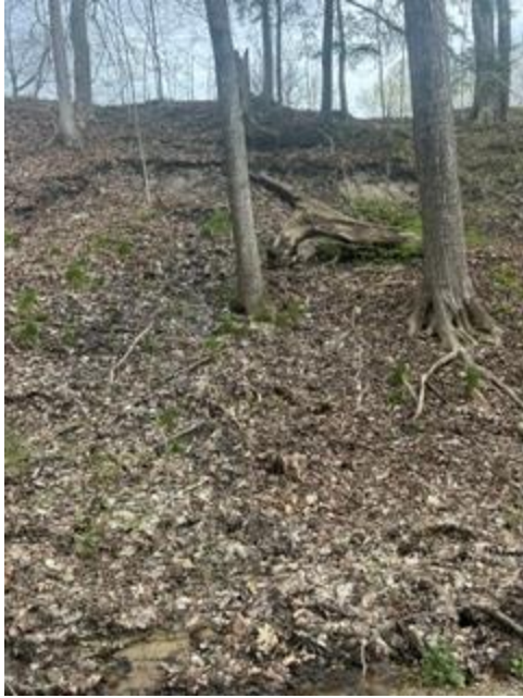
Large bank slump creating unstable bank condition
