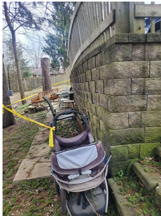
Precast Block Retaining Wall View looking North - April 17, 2026 (Site Location - see Figure No. 1)
