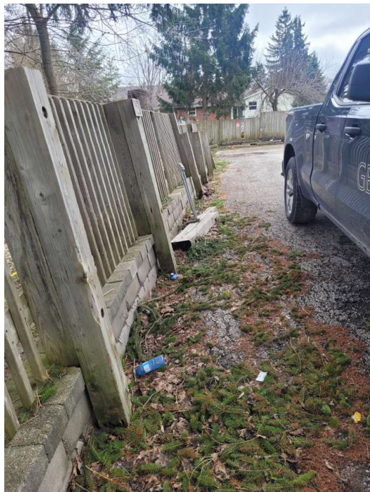
Precast Block Retaining Wall View looking South - April 17, 2026 (Site Location - see Figure No. 1)
